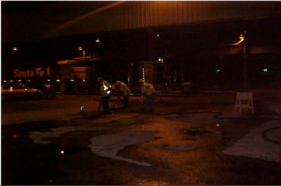
View Southwest - Vacuuming and applying absorbent to the spill area.
